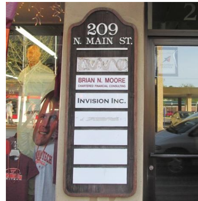
A directory sign at the main entrance can be used to identify all tenants
