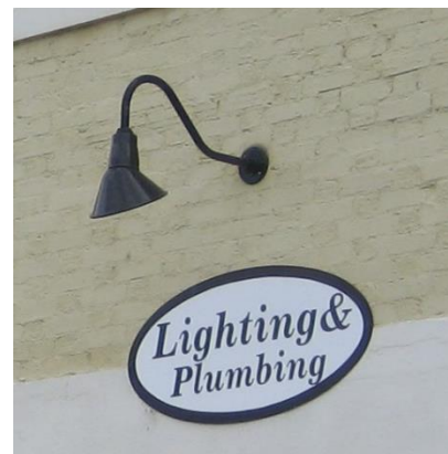
Sign illuminated indirectly with shielded light source
