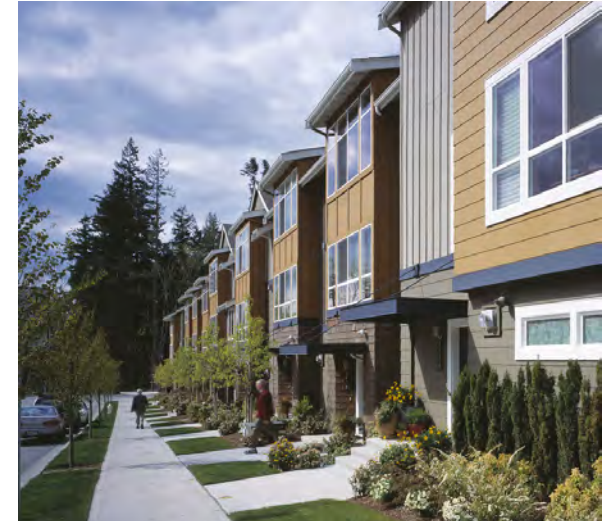
Vertical &amp; horizontal building articulation
