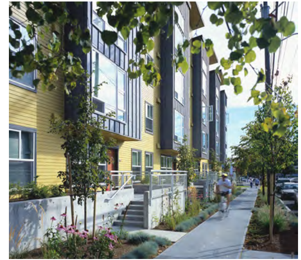
Entrances above the sidewalk
