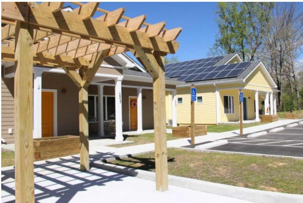
Grissom Lane Senior Housing, built to net zero energy standards meaning each home produces as much or more energy than it uses
