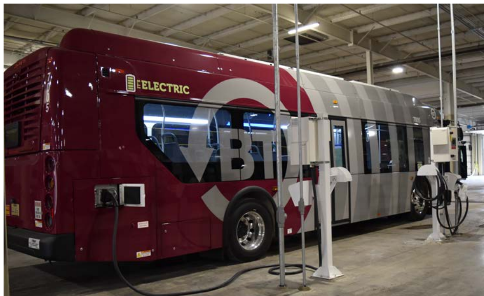
Blacksburg Transit electric bus charging
