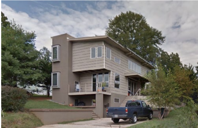
Charlottesville Internal ADU Credit: Design Develop LLC
