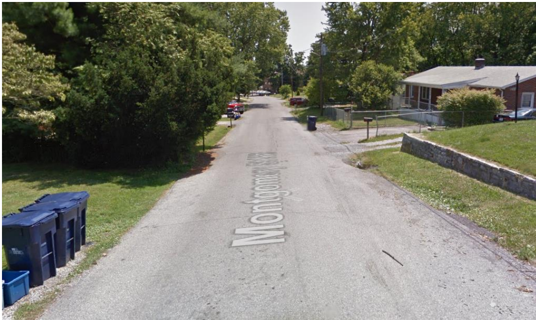
Figure 1. Example of Town Street with “roadside ditches and driveway culverts”, Google Street View.
