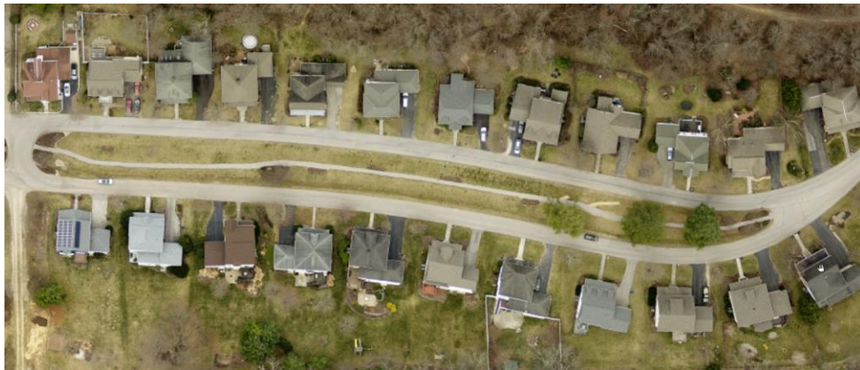
Figure 2. Median multi-use trail at VATC installed in lieu of sidewalks.
