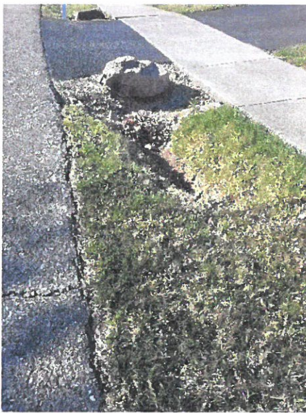
Driveway outlet. – ditch filled in
