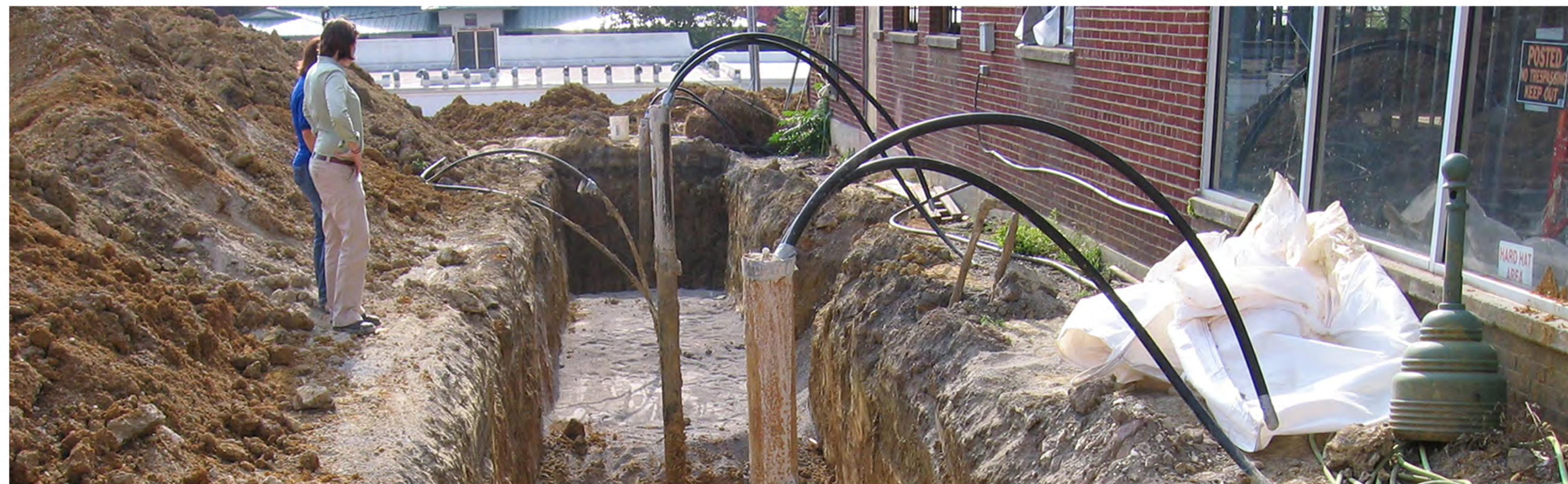
GEOTHERMAL WELL INSTALLATION IN PROGRESS
