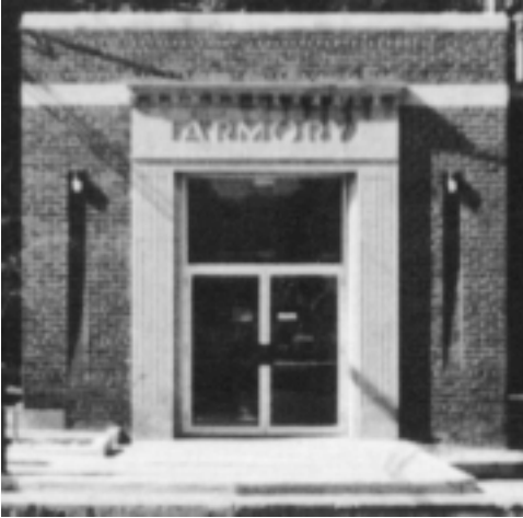
Lighting detail in a brick facade where graduated brick pockets frame the wall sconces
