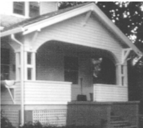
Corner porch detail with an open frame column enlarges the street view
