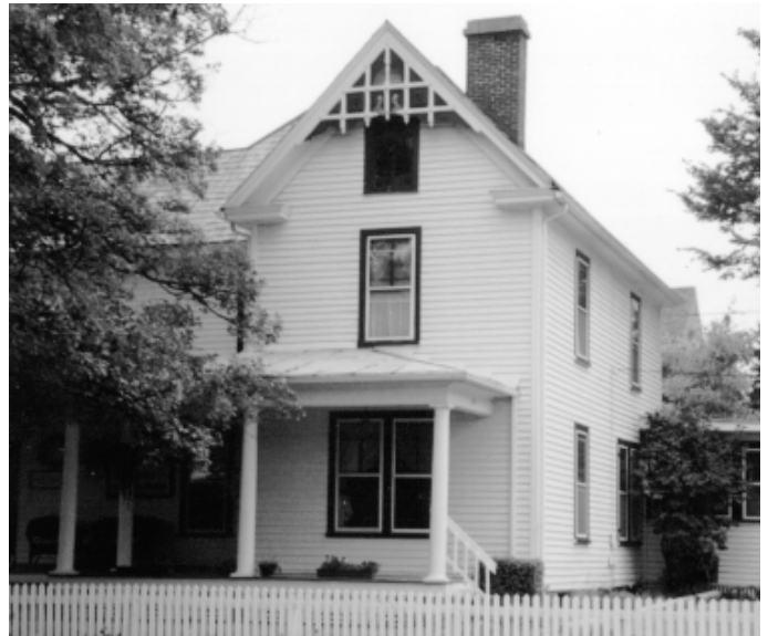
A house on Main Street is an example of a conversion to a business where the detail has been maintained
