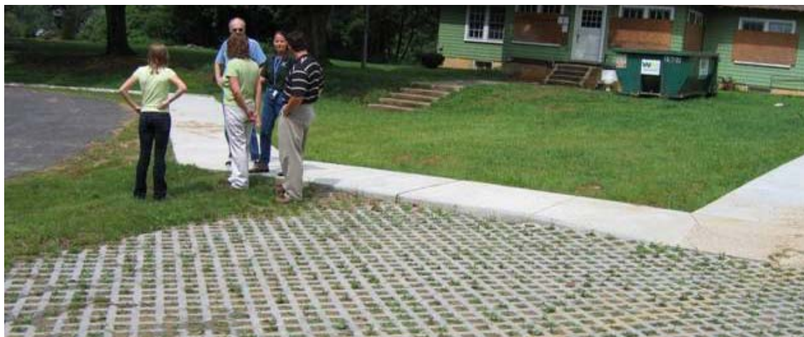
Grass pavers installed at Wong Park
