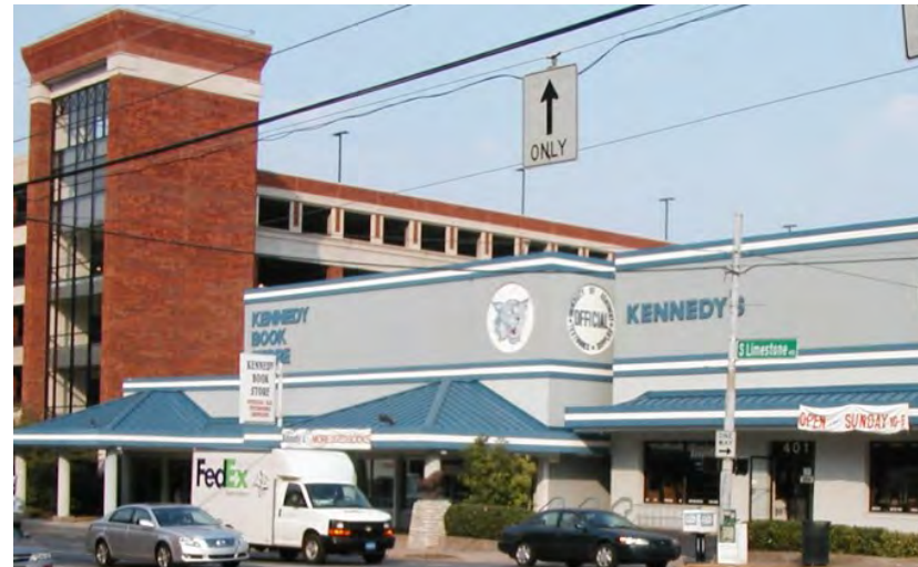
The South Limestone garage in Lexington services the University of Kentucky during weekdays, and a commercial district on the evenings and weekends.
