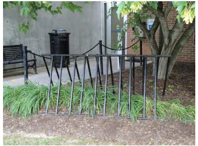
Photo 45: Municipal Building - North
