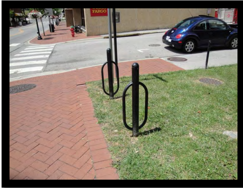
Bicycle parking in Town of Blacksburg
