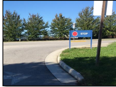
Install compliant MUTCD Stop sign
