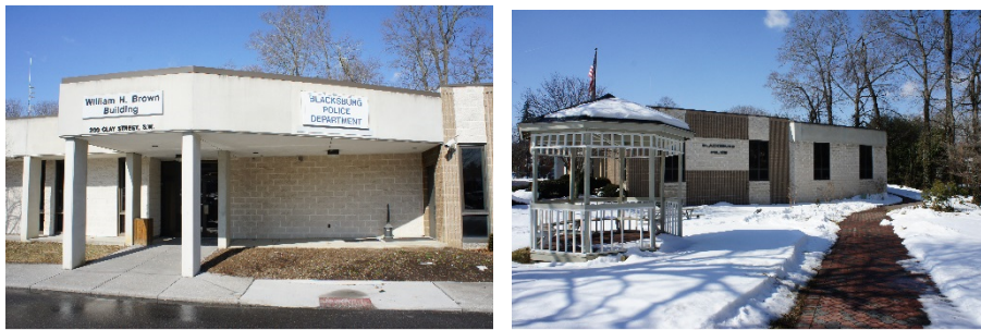
Existing Police Department
