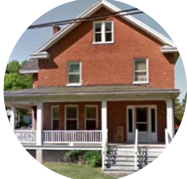
Homes with Architectural Character
