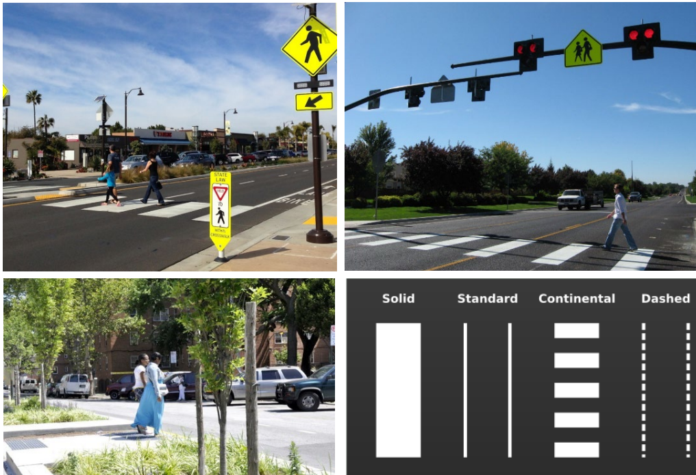
Examples of Rapid Flashing Beacon (upper left) and HAWK (upper right) crossing systems, pedestrian refuge island (lower left), and types of crosswalks (lower right).
