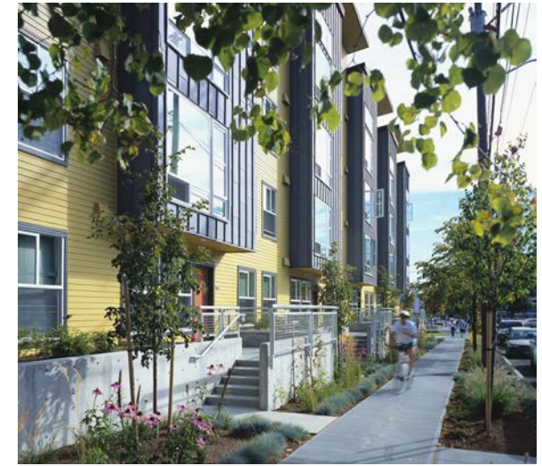
Entrances above the sidewalk
