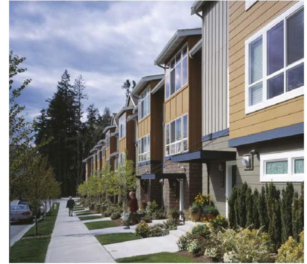
Vertical & horizontal building articulation
