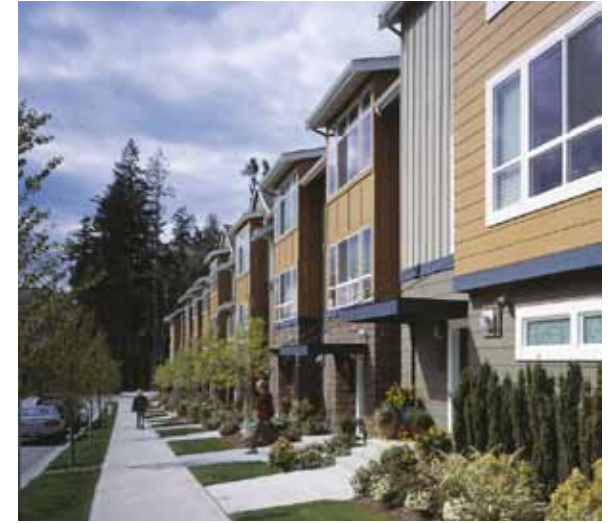
Vertical &amp; horizontal building articulation
