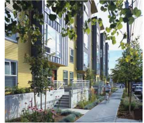
Entrances above the sidewalk
